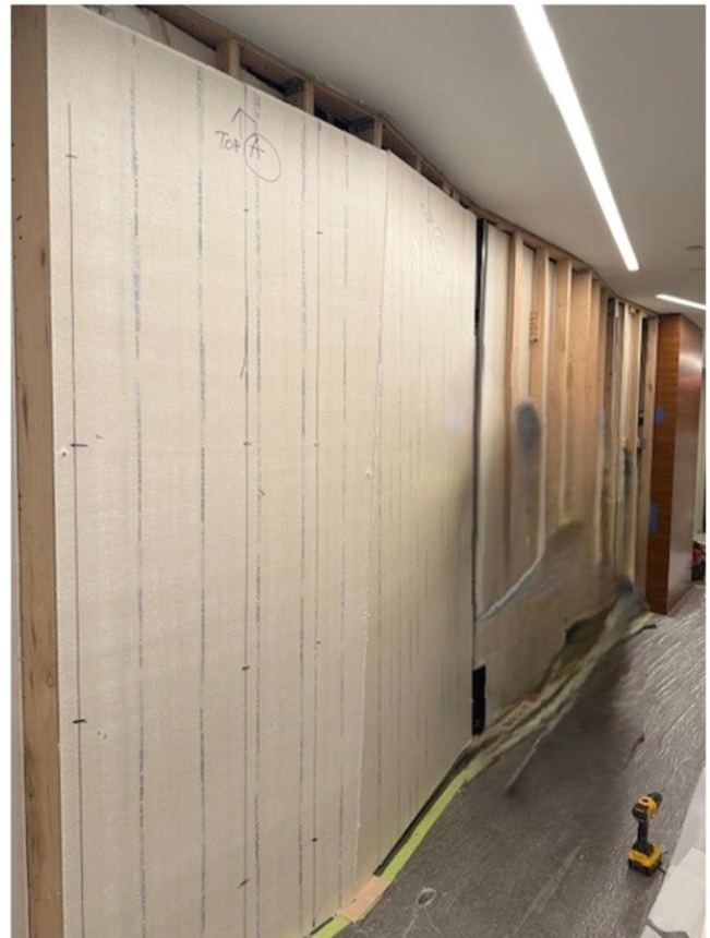
Above and Right: New UL 7 Concealed Ballistic Panels installed on new framing.
