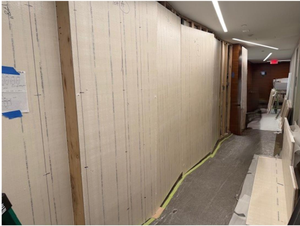
Above and Right: New UL 7 Concealed Ballistic Panels installed on new framing.
