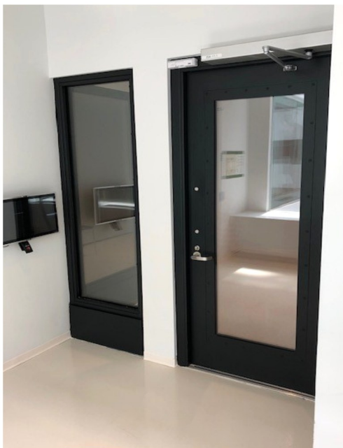
Ballistic, forced entry resistant door, incorporating automated door closure.
