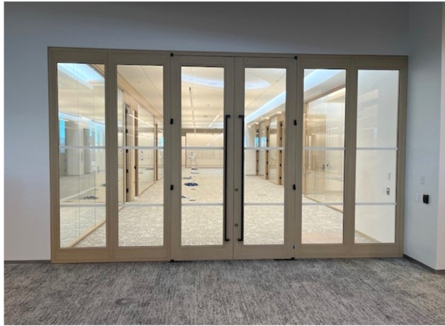
Full-light, wood clad , ballistic entry elevation.
